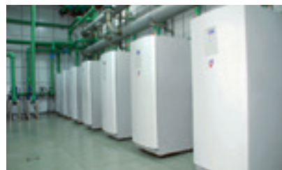
Seven Thermia Robust Eco units connected together.
